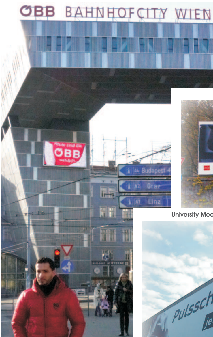
Austrian railway company "ÖBB" believe in the high quality of ACT videowalls and use them for the new railway station "Vienna West". At high level installed it can be readable from far away
