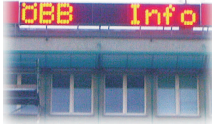
80cm character height, mounted on a roof
